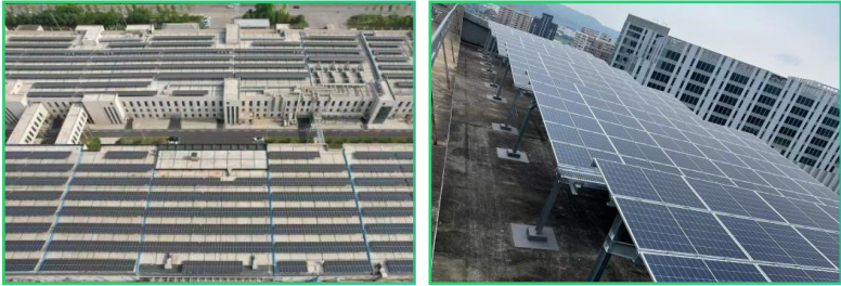
Energy Saving and Carbon Reduction Performance: Solar power installations at the Xuzhou and Taiwan plants began operation in 2024, actively demonstrating FOXLINK’s commitment to achieving carbon emission reductions.
