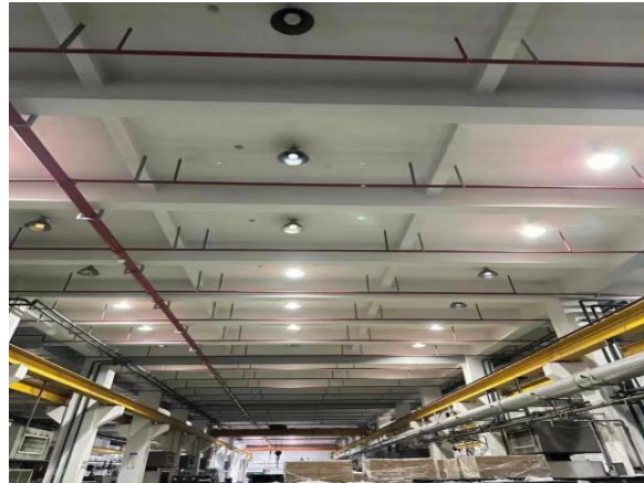
Installation of fire sprinkler systems
